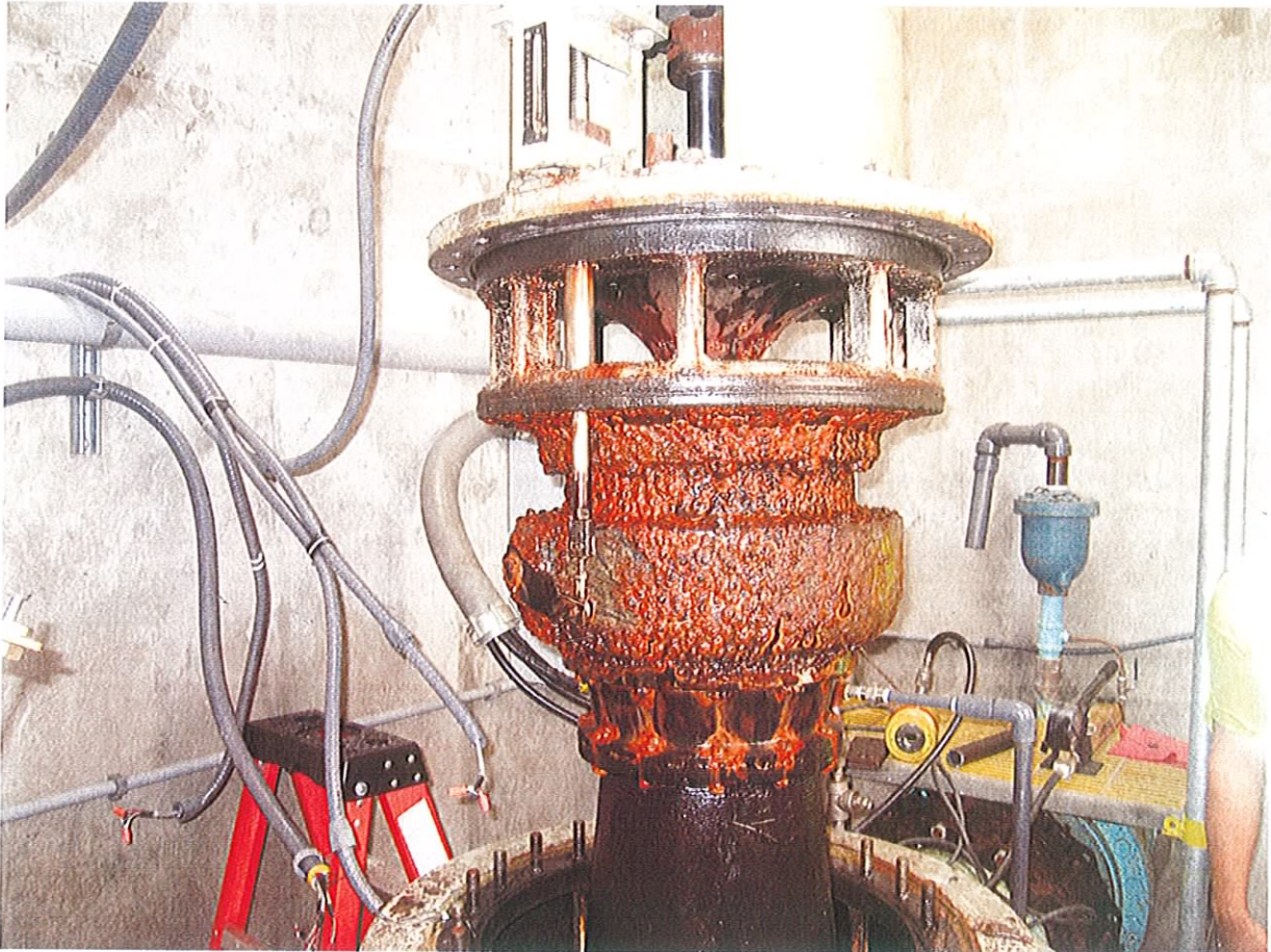
The hydro-electric turbine being removed for preventative maintenance.
